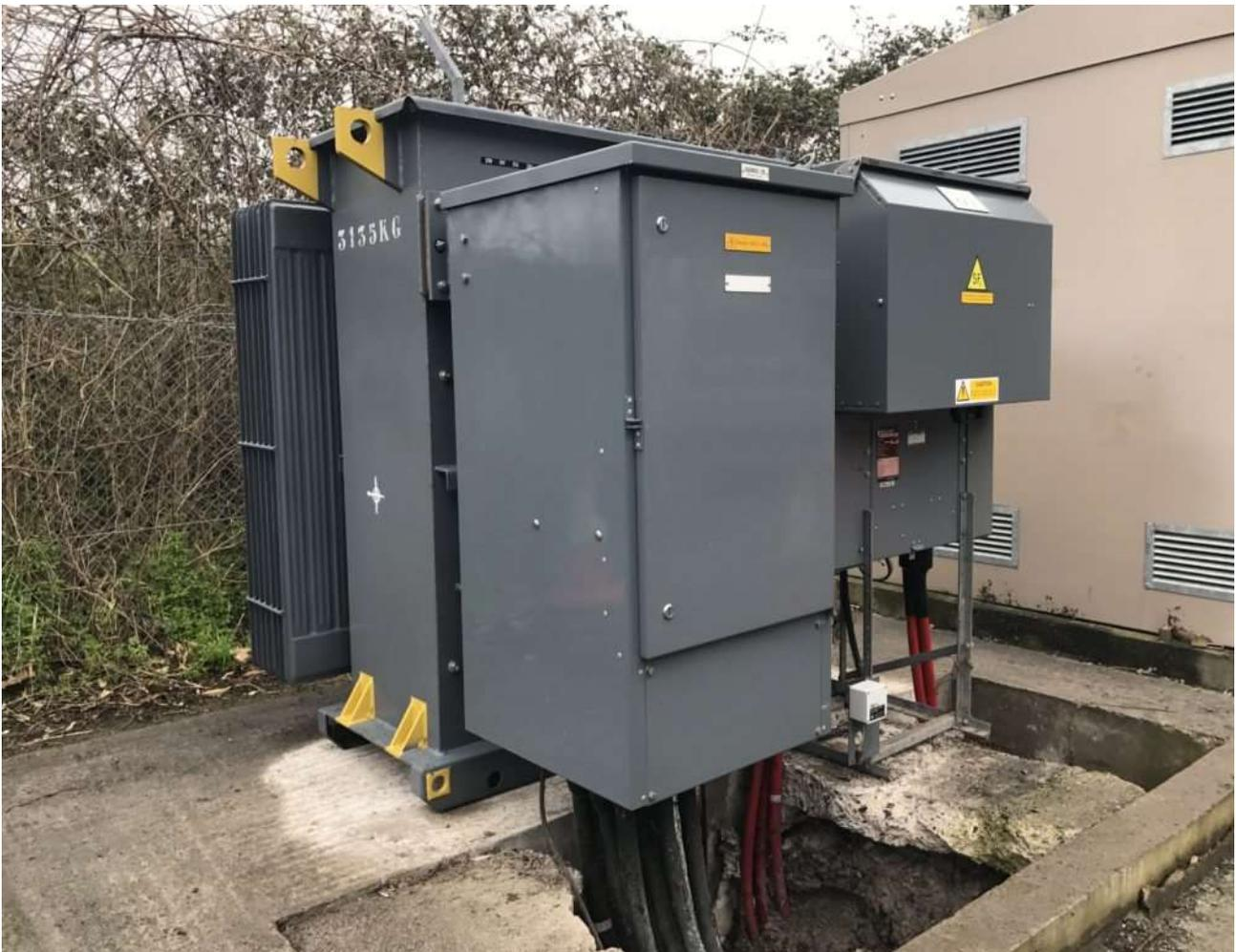
*Figure 7: Indicative example of an 11kV UDE*
